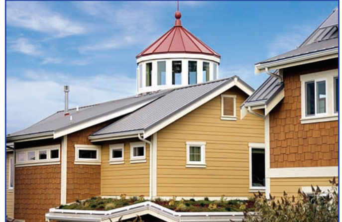
Going Green at the Beach home meets or exceeds the requirements of six major and prestigious Green Building programs. Icynene helped the home achieve LEED Gold Status.
