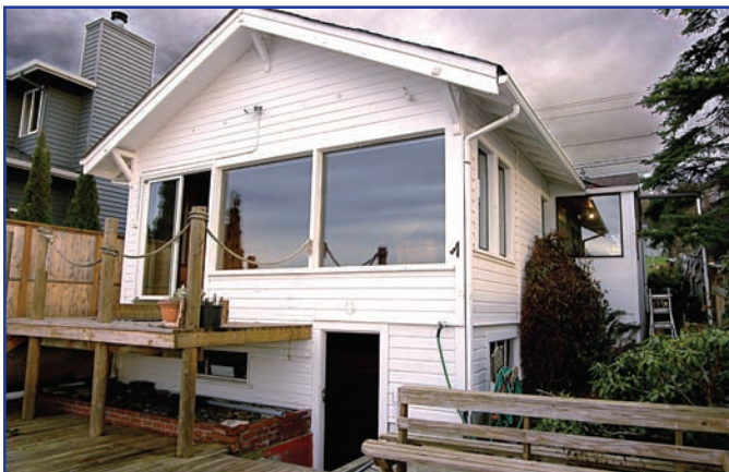
The 100-year old home, originally constructed in 1907, was in a state of disrepair; therefore, it was deconstructed and rebuilt.
