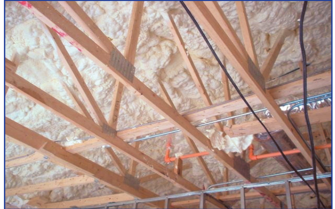
Incorporated with a properly sized HVAC system, Icynene minimizes the potential for condensation and related problems like mold growth.
