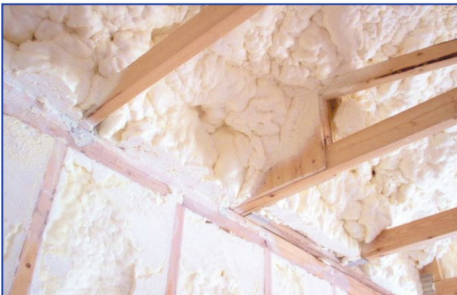
Icynene softly expands to 100 times its initial volume to completely fill all gaps and crevices that compromise airtightness. Areas that are considered difficult to insulate with conventional insulations are no obstacle for Icynene. Attics, ceilings, and walls can be quickly and easily insulated.
