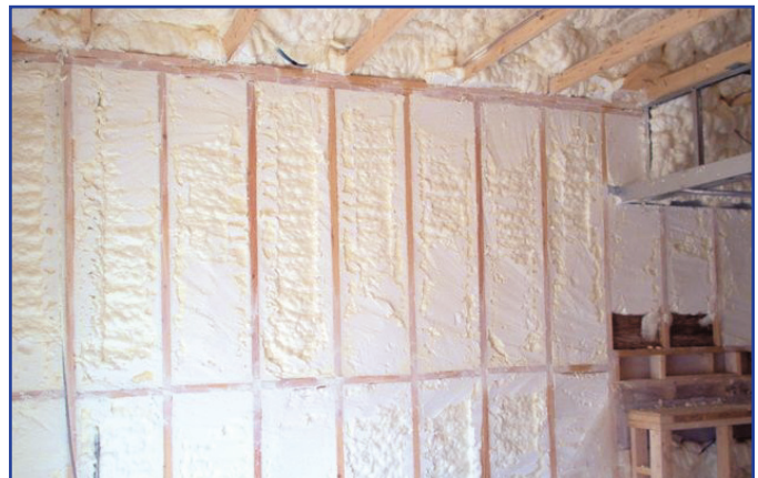
With Icynene sprayed into the exterior wall cavities, the sound from the quarry 2 miles away will be minimized, thereby ensuring the comfort of the residents and staff of the Home.
