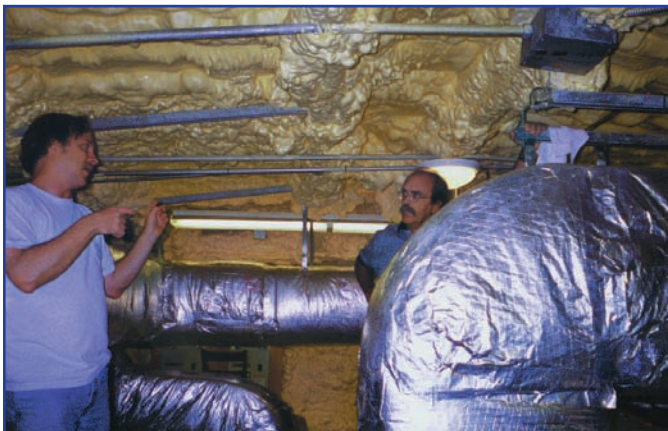
Wendell Porter of the University of Florida demonstrates, on a June day, how Icynene keeps the unconditioned mechanical room at a comfortable temperature.
