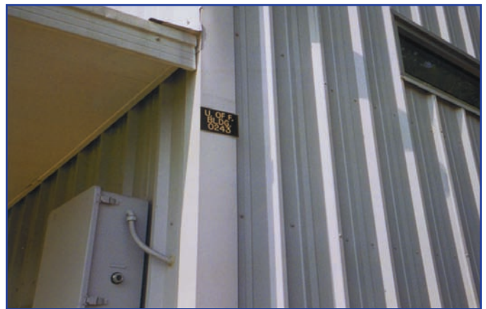
The building utilized standard corrugated steel panel construction.
