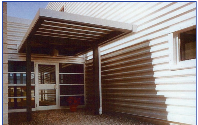
ICYNENE LD-C-50™† insulation and air barrier was installed because it contributes to the achievement of LEED credits, such as energy performance and thermal comfort.
