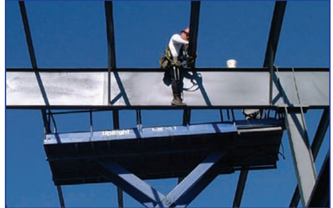
In keeping with the philosophy of green design, all concrete and metal scrap was recycled.
