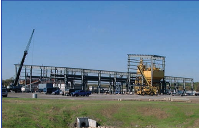
Formerly the site of a steel sintering plant, this designated Brownfield site has been revitalized to LEED standards and now features a healthy, productive workplace for Castcon employees.
