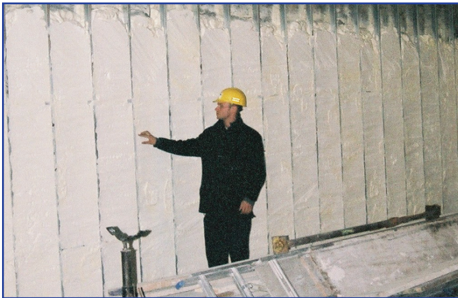
Penta Protective Coatings, Icynene Licensed Dealer in West St. Paul, Manitoba, sprayed Icynene into the exterior walls of the building to protect the shell from a major source of energy loss – air leakage.
